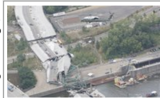
(AP) Marine One, carrying President Bush, top, flies over the collapsed Interstate 35W bridge over the... Full Image
